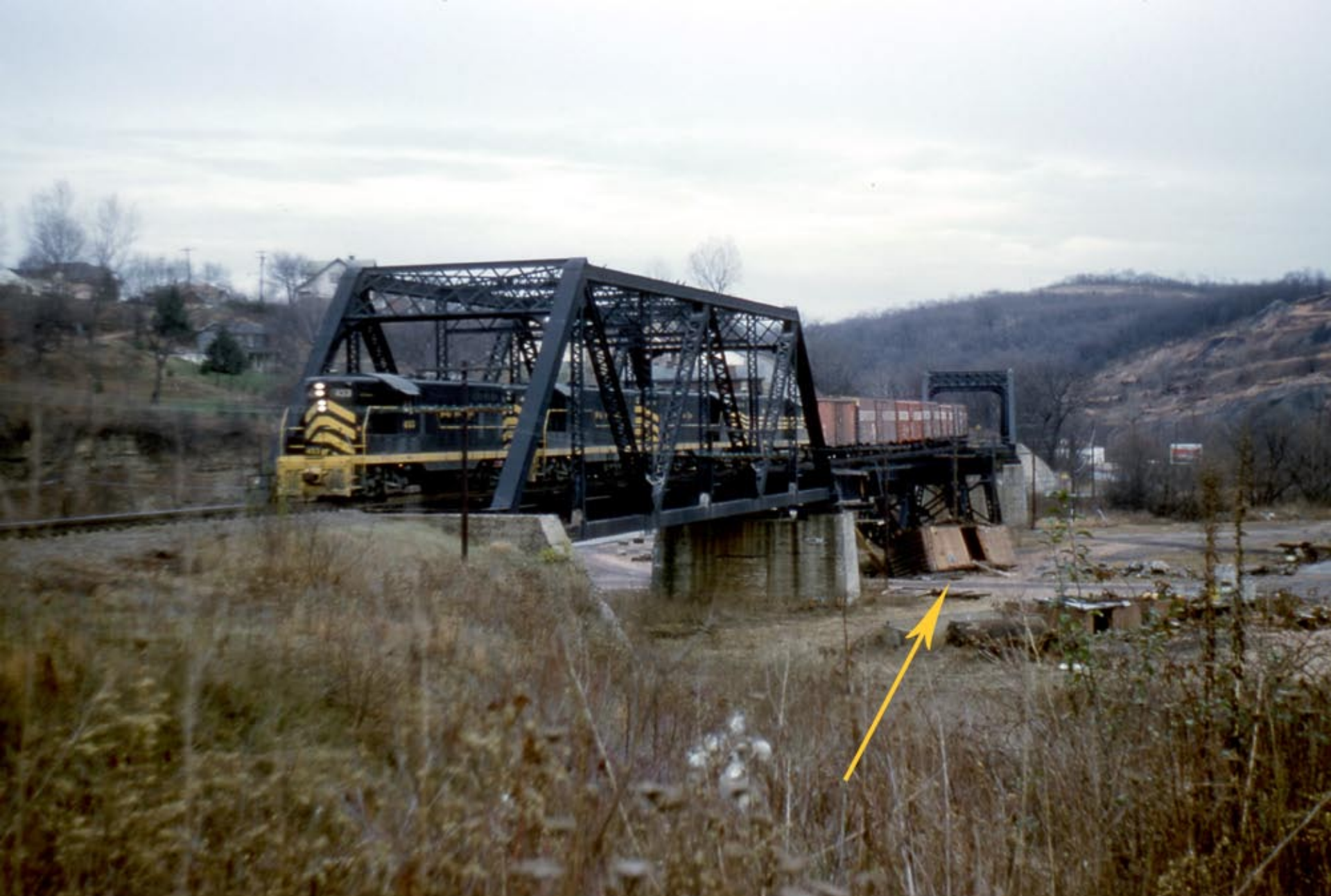
The Sygan bridge showing the previous derailed refrigerated box car MRBX 276 at MP 62.02
